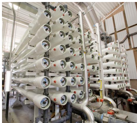
Reverse Osmosis membranes – similar to those at Zone 7's Mocho Demineralization Facility – would provide highly treated recycled water for injection into the Main
