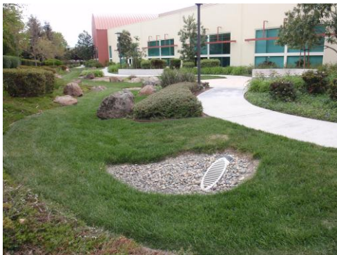
Drain rock is used to prevent erosion of this vegetated swale at Zone 7 Water Agency's office building – drain rock can also enhance recharge if placed over permeable areas of the groundwater basin.
