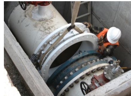
Construction of El Charro Pipeline in 2009
