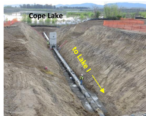
Lake I to Cope Lake Intertie (completed in May 2014)
