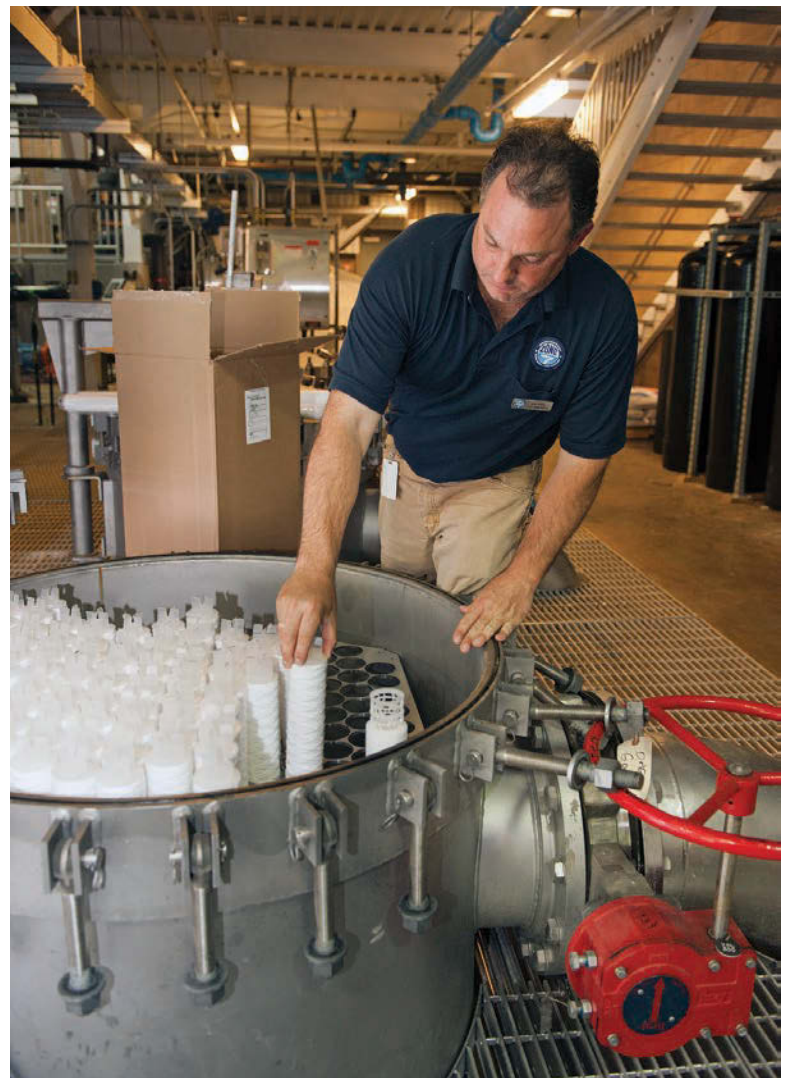
Plant operator 3 John Brixie changes the cartridge filters (Parker Hannifin) on the reverse osmosis prefiltering system.
