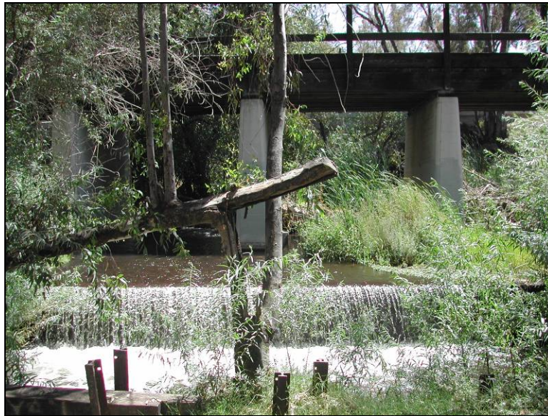
Figure 3-28: Railroad Crossing Footing at Stanley Boulevard
