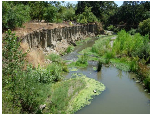
Figure 3-17: Bank Erosion along ADLL Immediately Downstream of the Verona Avenue Footbridge
