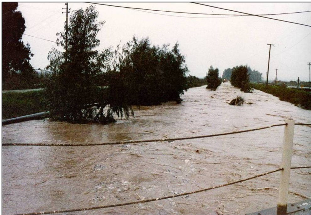
Figure 3-2: 1998 Flood Waters in Arroyo Mocho at the El Charro Road Crossing
