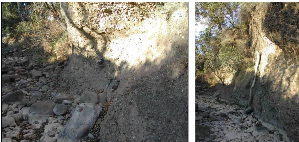
Figure 3-18: Bank and Toe Erosion in Sinbad Creek
