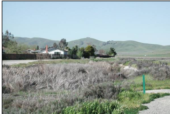
Figure 3-11: Sediment Deposition and Vegetation Debris in Reach 1 along Altamont Creek
