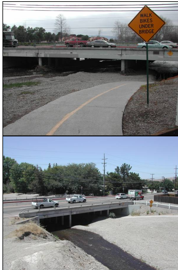
Figure 3-14: Gravel Deposits along Arroyo Mocho at Holmes Street Bridge in Reach 3
