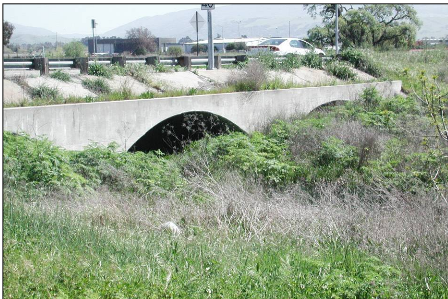
Figure 1-8: Sedimentation along Arroyo las Positas near Airway Boulevard
