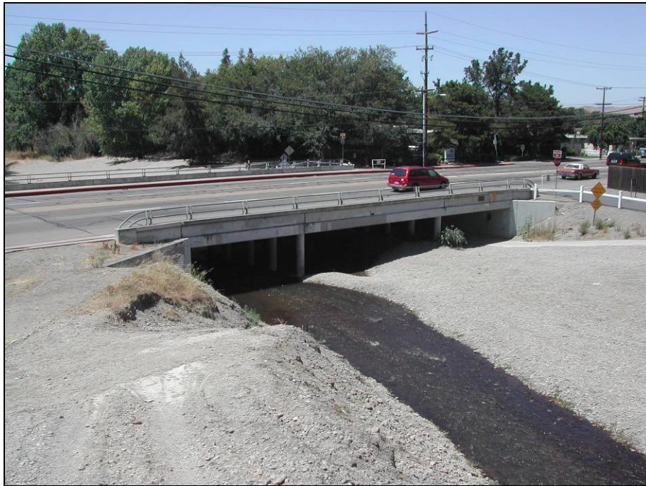
Figure 1-9: Sedimentation along Arroyo Mocho at Holmes Street Bridge
