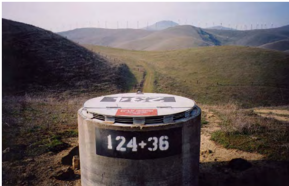
Example of finished vault structure
