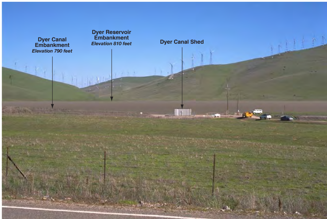
Dyer Reservoir from public road at 3226 Dyer Road – Constructed View
