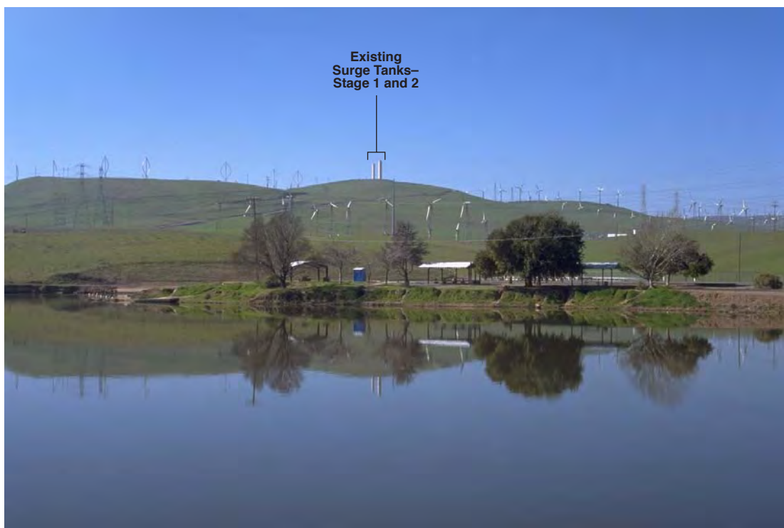
Surge Tank from Bethany Reservoir Recreation Area – Existing View
