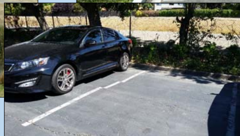
CRACKING AND DIFFERENTIAL VERTICAL OFFSET - Concentrations Near Large Exposed Unpaved Areas, Slopes (e.g. Canal Banks) In Areas With Expansive Soils, +/- Rows of Trees
