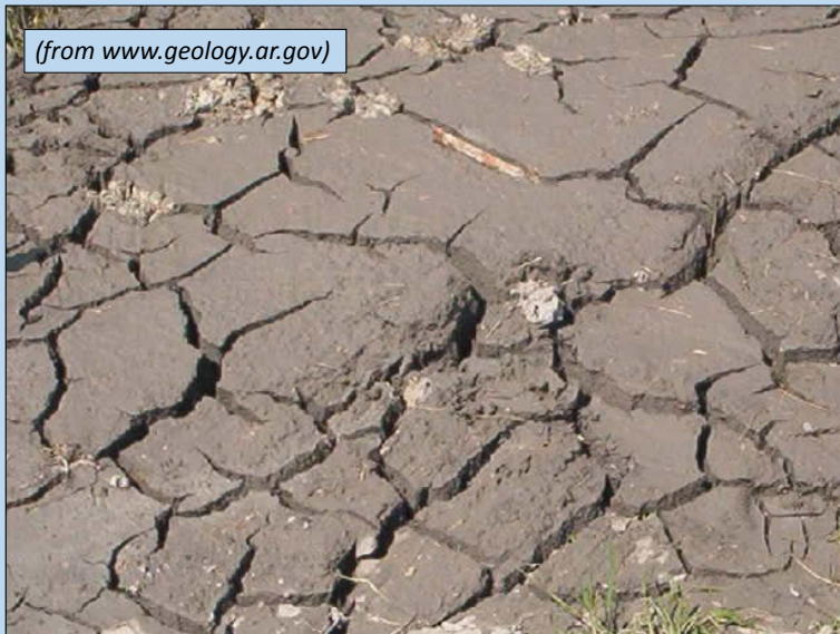
Expansive Soil Desiccation Cracks
