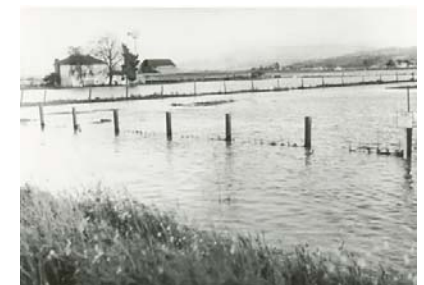
Flooding near Mohr Avenue, Pleasanton
