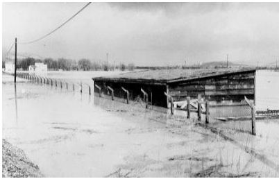
Flooding near Hopyard Road in Pleasanton
