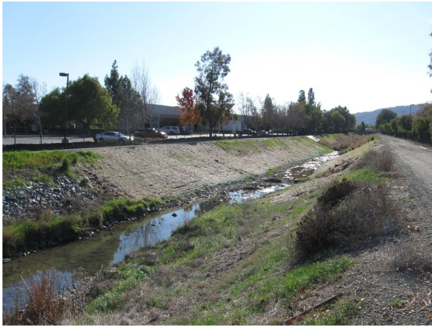
September 2011: Completed work including hydroseeding.
