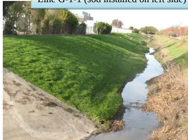
Line G-1-1 (sod installed on left side)
