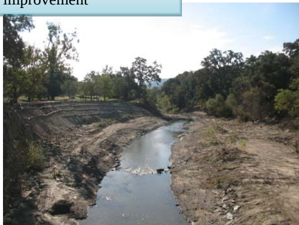
Stream bank stabilization improvement
