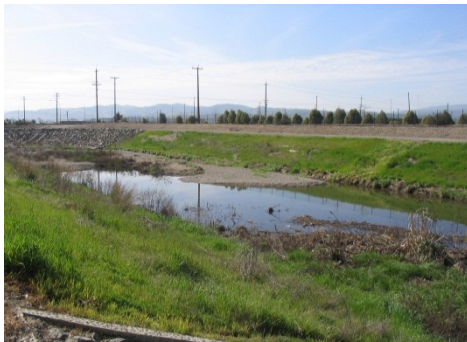
Figure 4. The sedimentation basin near Isabel Ave. requires periodic maintenance (removal of accumulated material).
