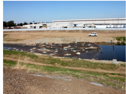
Figure 7. Example of a recently constructed roughened channel in Stockton (note lattice structure), without vegetative enhancements
