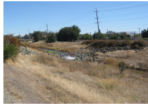
Figure 5. One of the four existing grade control drop structures to be removed / modified.
