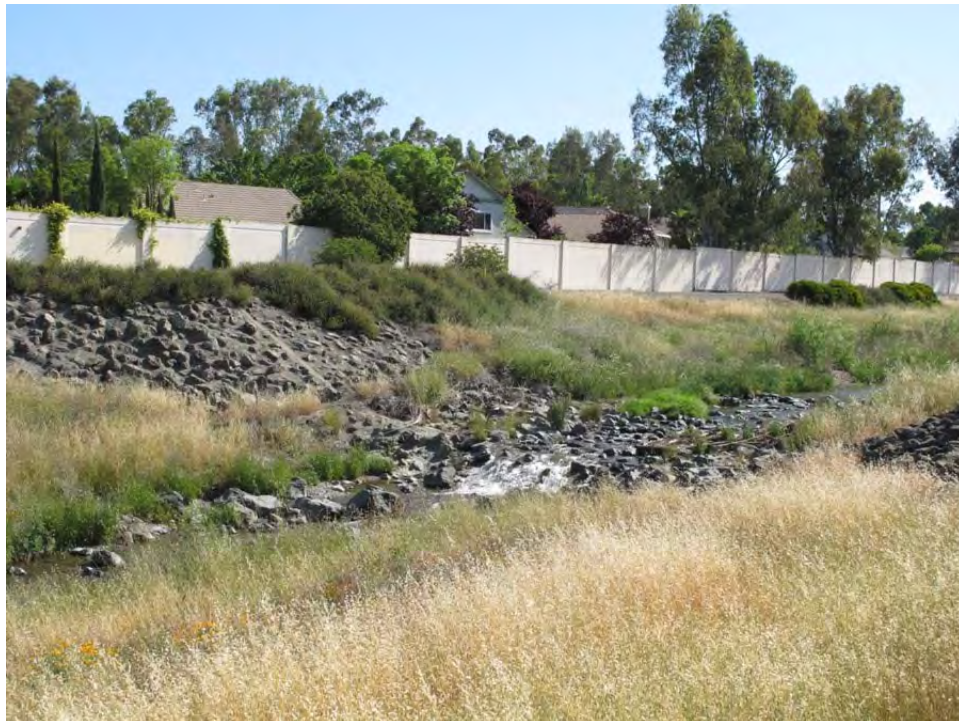
Source: ESA Stanley Pilot Project. 201459.06 Figure 4 Representative Photographs of Grade Control Structures Identified for Removal
