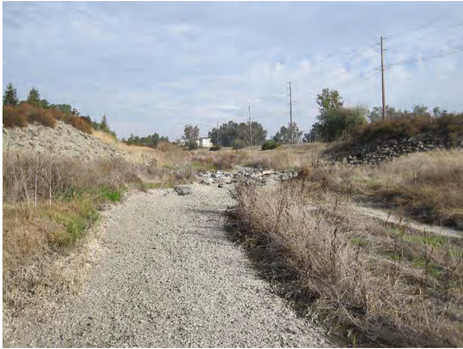
Photo 3: View of the eastern-most grade control structure facing east. Photo shows instream wetlands and channel of Arroyo Mocho. (November 15, 2012).
