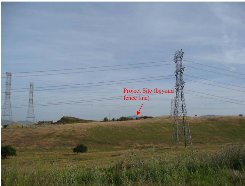
Photo 6-2. View of the DVWTP southern boundary from near the highest trail location in Sycamore Grove Park. From this location, some of the proposed solar panels will be in partial view at most times of the day.
