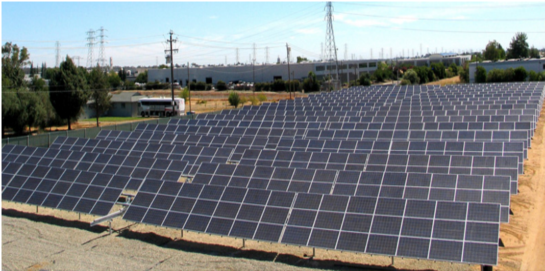
Figure 3. Example of a Single Axis Photovoltaic System
