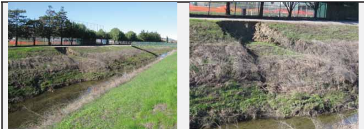
Photo Set 4: Site #4 (Line J)
