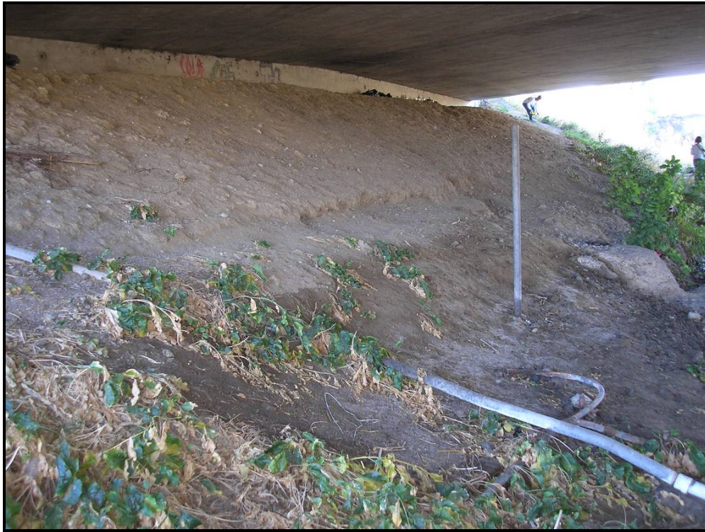
Photograph 2-3. Existing South Channel Bank
