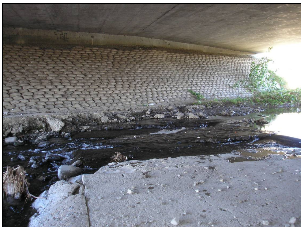
Photograph 2-2. Existing North Channel Bank
