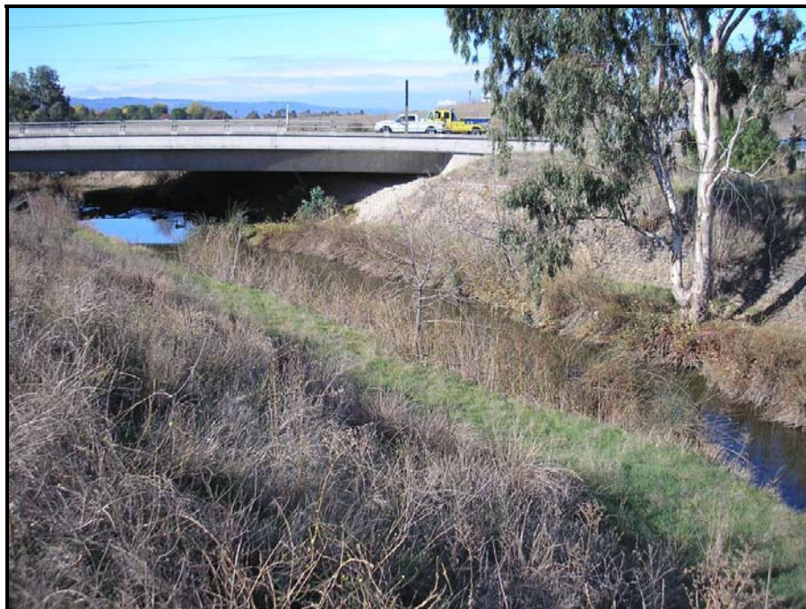
Photograph 2-5. Lateral Access from Top of Stream Bank to Weir Site
