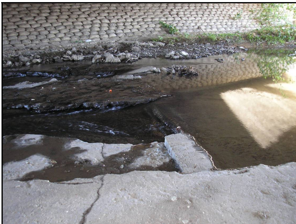
Photograph 2-1. Existing Concrete Pad and Sill
