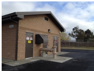
Chain of Lakes Well No. 5 (completed in October 2014)
