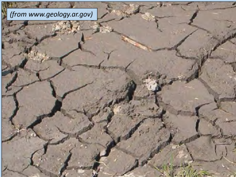
Expansive Soil Desiccation Cracks
