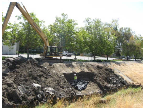
Chabot Canal Construction Begins
