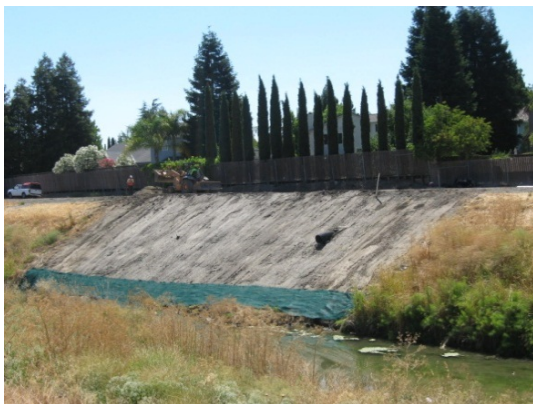
Completed Arroyo Mocho Repair
