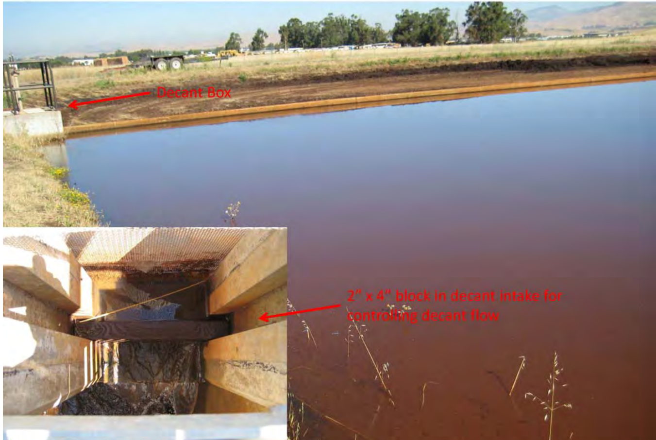
Figure 2 – Sludge where 1 -2% solids settle and water on surface goes to decant box
