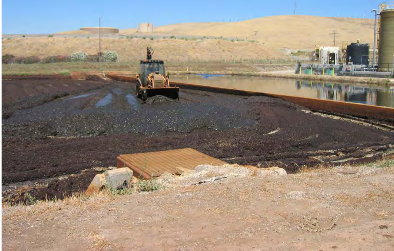
Figure 4 – Bobcat with tiller to agitate or churn up caked surface so that sludge beneath gets exposure to sun.
