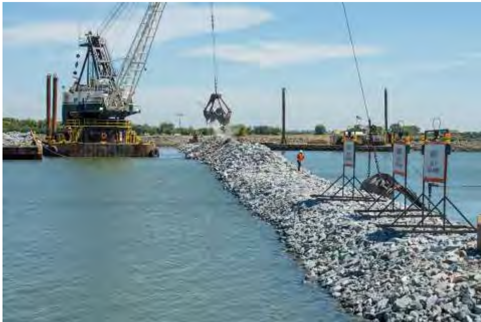
Completing Delta rock barrier (photo by DWR)
