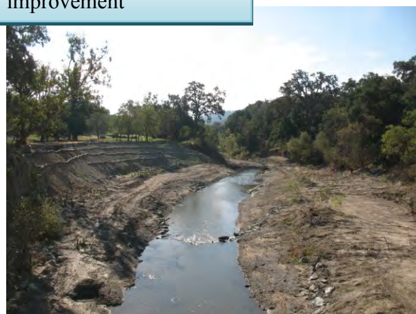
Stream bank stabilization improvement
