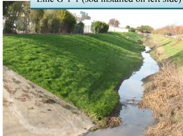
Line G-1-1 (sod installed on left side)
