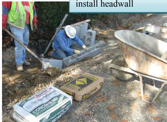
Alamo Creek at Line J-1 install headwall
