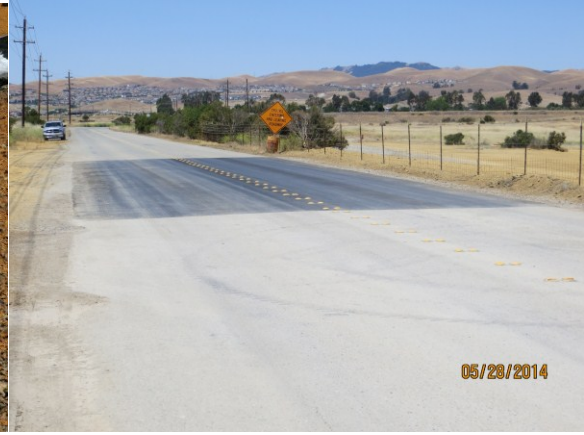
Repaired Haul Road Section
