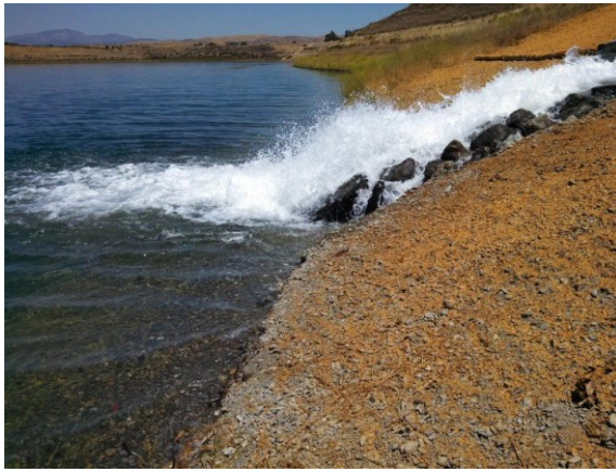
Lake I Outfall (Discharge ~ 8 mgd)
