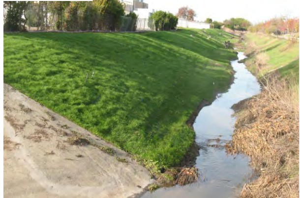
Line G-1-1 (sod installed on left)
