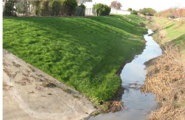
Line G-1-1 (sod installed on left)
