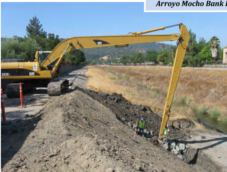
Arroyo Mocho Bank Repair
