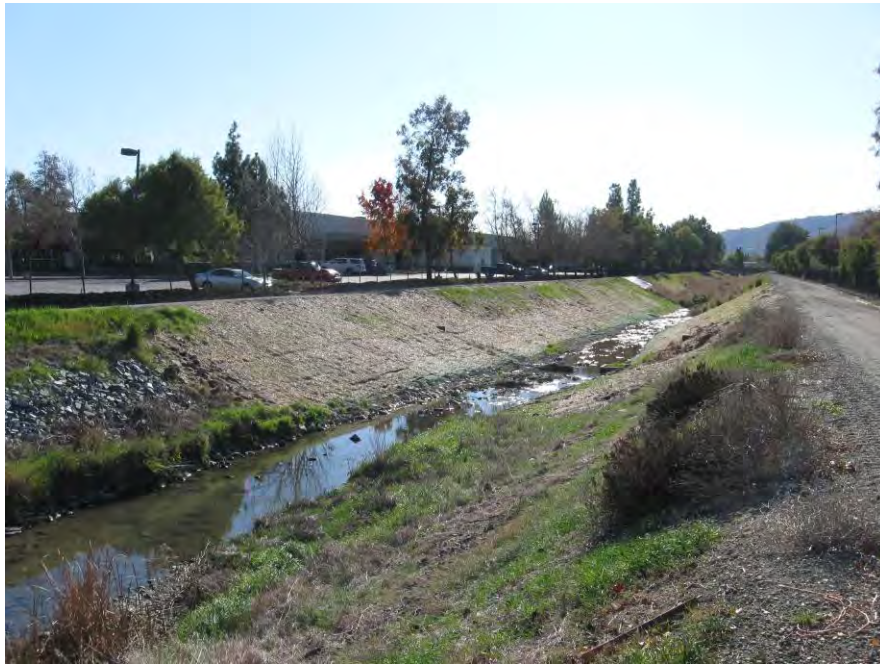
September 2011: Completed work including hydroseeding.
