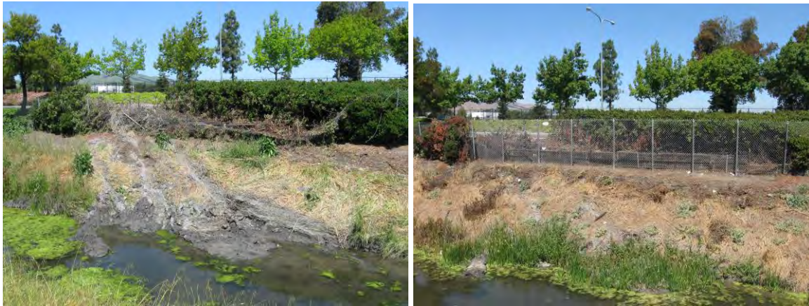
Line G-1-1 in Pleasanton: The fence adjacent to Stoneridge Dr. was damaged due to an out of control vehicle. Calco Fencing contractor came in and repaired the fence to its original state.
