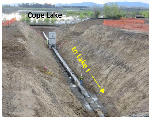
Zone 7 is firming up groundwater supplies for this summer by constructing a pipeline that will recharge mining discharges back into the groundwater basin.
