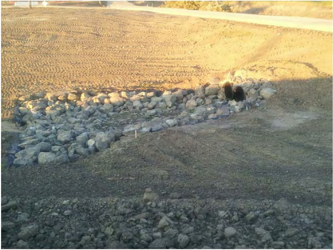
Temporary outfall from golf course into Southern Conveyance Facility.
