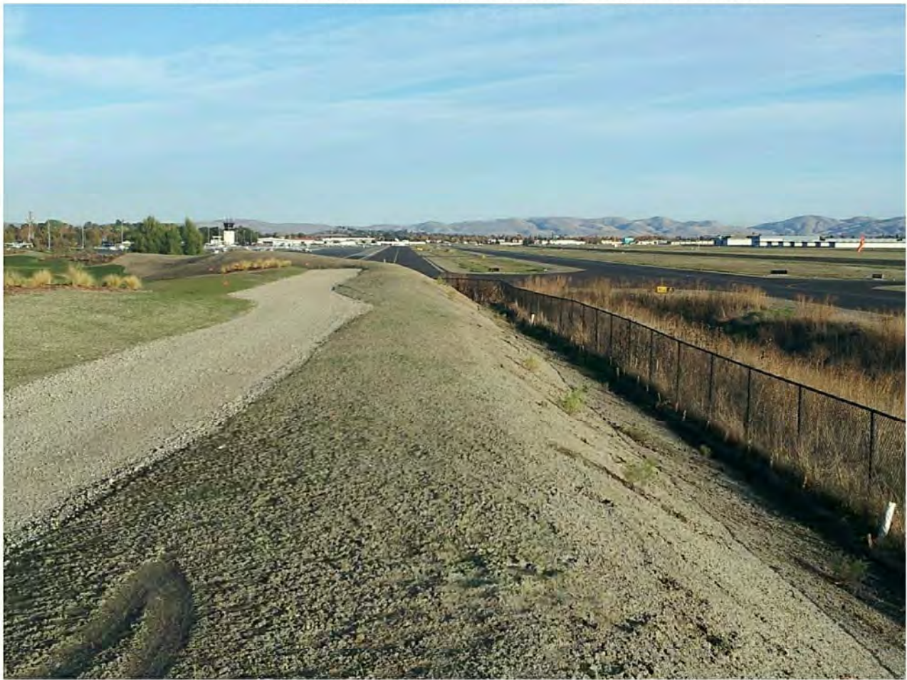
Looking eastward along berm ridge between Golf Course and Airport.
