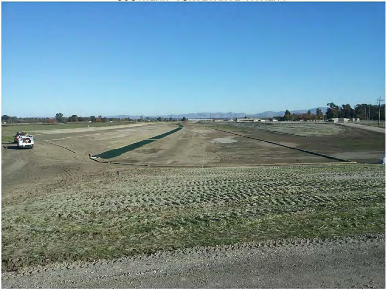
Looking eastward from northwest corner of Southern Conveyance Facility.
