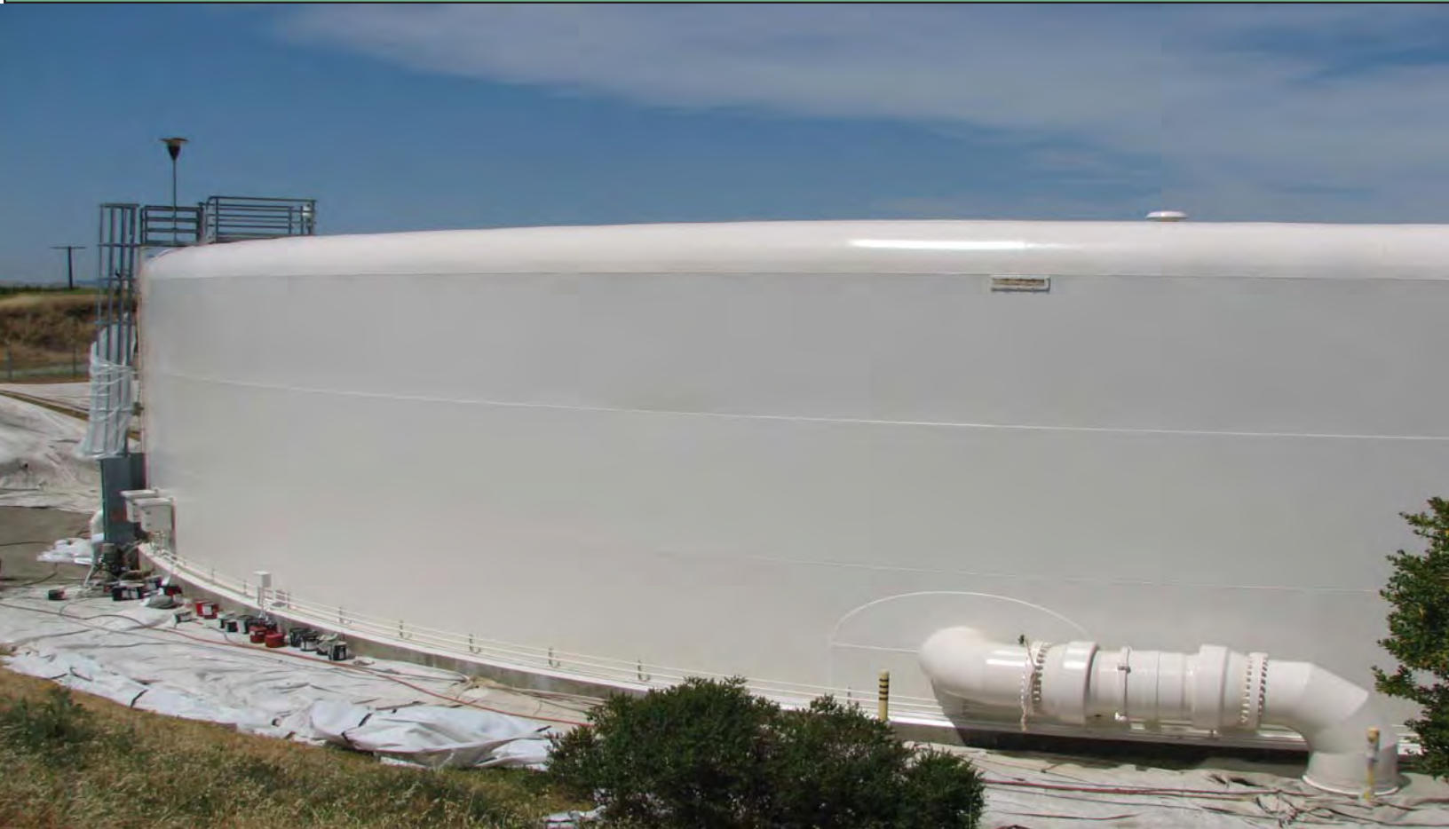
A Recently Recoated Clearwell at DVWTP
